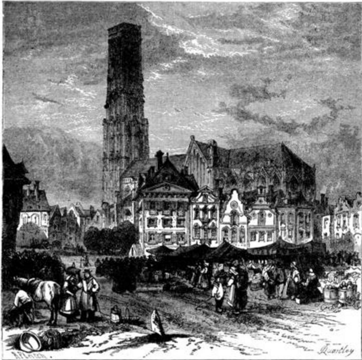
VIEW IN MECHLIN.
